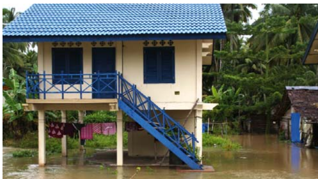
Reconstruction: earthquake resistant and flood proof houses built within a GRC project in Indonesia after the 2004 tsunami.
